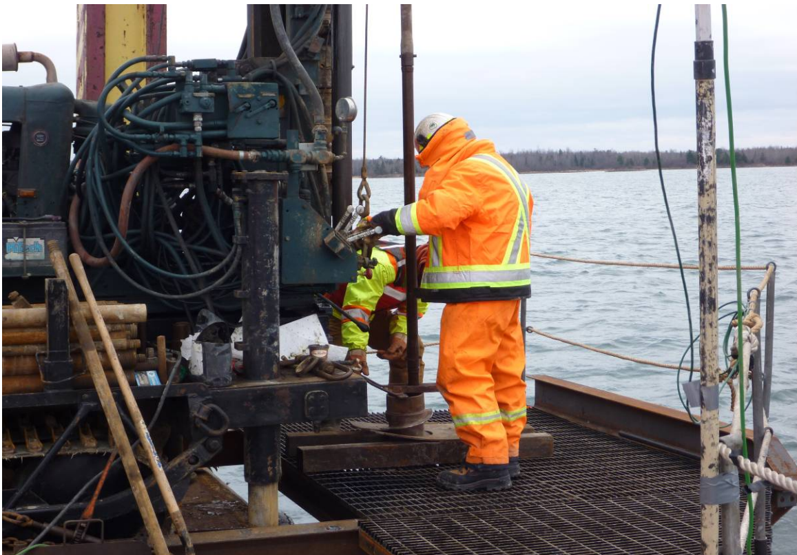
Photograph #4 – Advancing borehole
