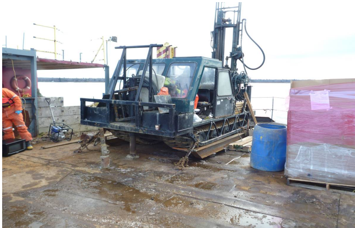
Photograph #2 – CME 850 drill rig mounted to 100 tonne capacity barge
