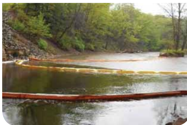
Containing a spill on Bronte Creek, a Lake Ontario tributary. (Ministry of the Environment)
