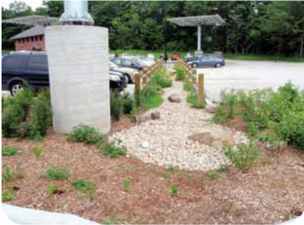
A bioretention area reduces pollution from parking lot stormwater at the Earth Rangers Centre in Vaughan. (Toronto and Region Conservation Authority)
