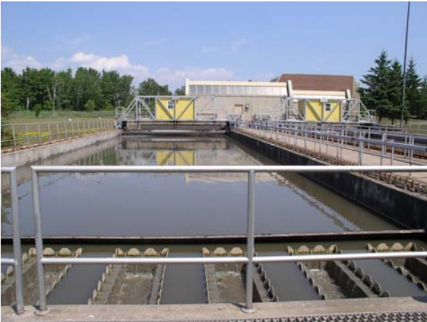
Figure 6.2. View of the West End Plant.
