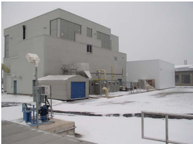
Figure 6.1. View of Sludge Dewatering Building.
